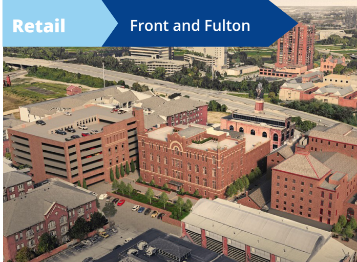
New mixed-use development in Brewery District that features office, apartments, a parking garage and 50,000 square feet of retail space.
